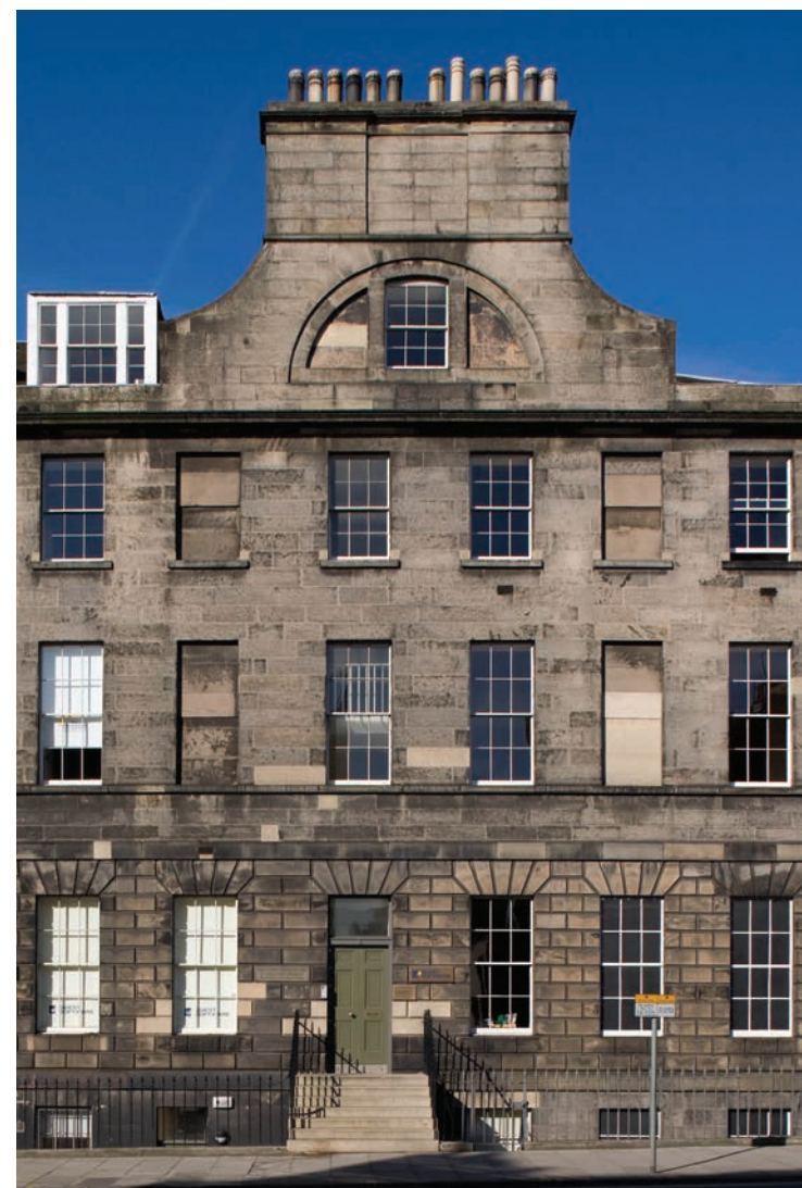
South Charlotte Street, Edinburgh. The blind openings are detailed with cills and a meeting rail to maintain the symmetry of the architectural elevation. There are chimney flues behind them within the walling.
