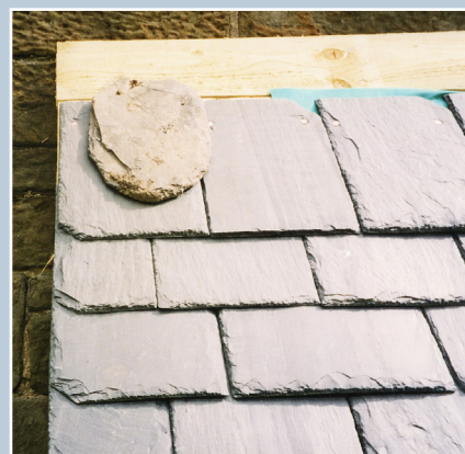
Sample panel prepared to ensure appropriate grading and random widths in the laying of new slate, with a fire-damaged Perthshire slate from Morgan Academy, Dundee.
